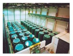
Figure 53: Storage in CASTOR<sup>®</sup> casks on the Dukovany nuclear power plant site (Czech Republic)
