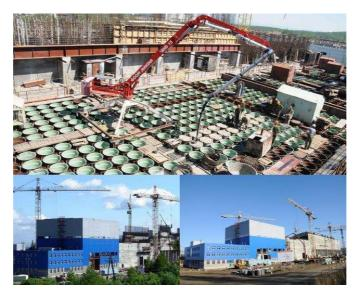
Figure 63: Photos of construction of the vaults and the centralised storage facility on the MCC site (Zheleznogorsk - Russia)
