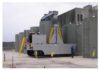
Figure 32: Photo of a storage facility using the HI-STORM 100 concept
