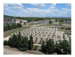
Figure 35: Storage facility on the Embalse site (Argentina) using AECL's concrete silo
