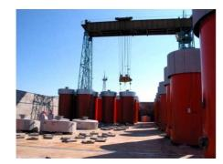
Figure 54: Storage in CASTOR<sup>®</sup> casks on the Ignalina nuclear power plant site (Lithuania)
