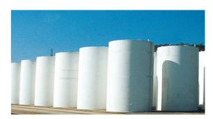
Figure 36: Storage facility on the Wolsong site (South Korea) using AECL's concrete silo
