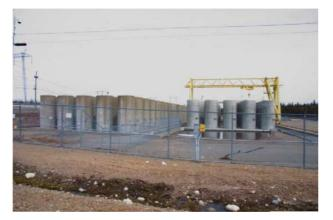
Figure 33: Storage facility on the Point Lepreau site (Canada) using AECL's concrete silo
