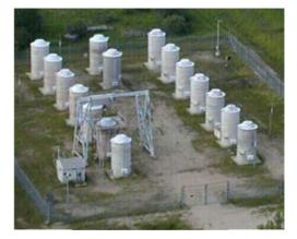
Figure 34: Storage facility on the Whiteshell site (Canada) using AECL's concrete silo
