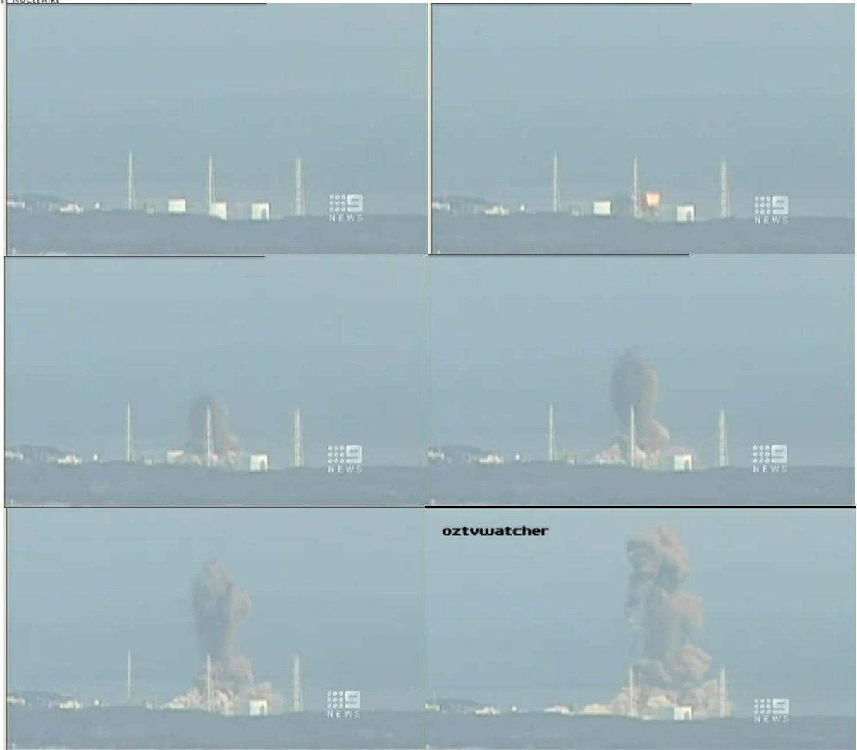
Figure 5-11 - 11:01 am on March 14: explosion in reactor building 3
