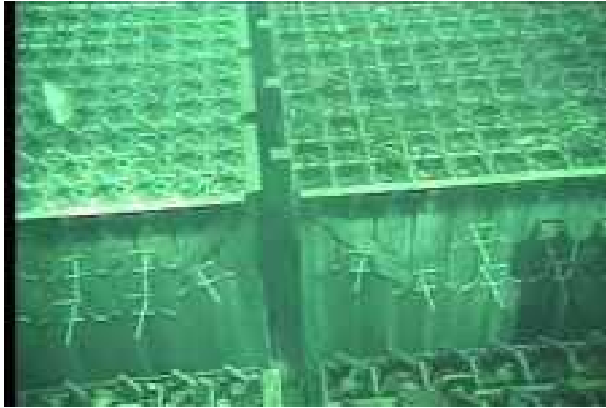
Figure 5-14 - Spent fuel storage racks in pool 4 after the accident (source: TEPCO)
