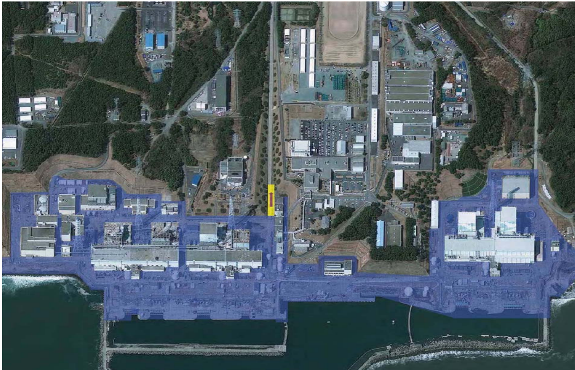
Figure 5-2 - Area inundated after the tsunami
