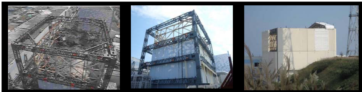
Figure 5-22 - Construction of the cover around the reactor 1 building
