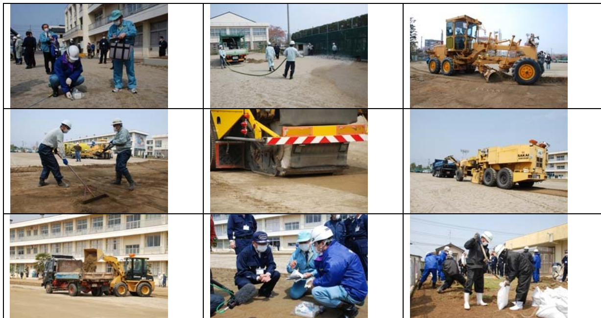
Figure 7-4 - Stages of surface stripping in schoolyards
