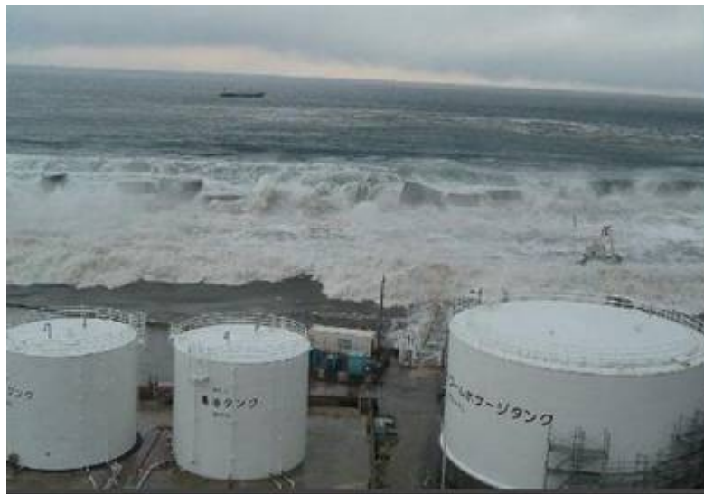
Figure 3-7 - Submersion of seawall at the Fukushima Dai-ichi site (source: TEPCO)
