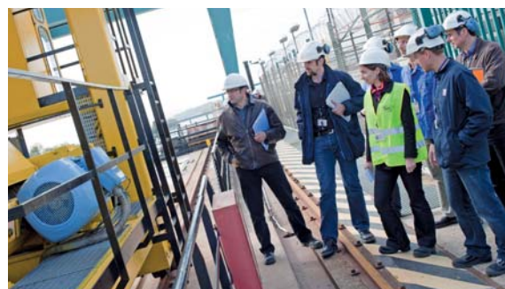
ASN-IRSN inspection of the cooling water pump station at the Cruas plant (Ardèche).
