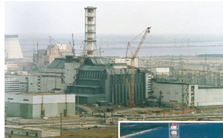
Chernobyl power plant. If the sarcophagus were to collapse, radioactive dust would be placed in suspension and could recontaminate the vicinity of the site.
